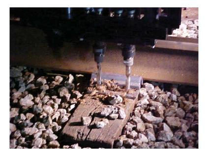
Four drills per workhead allow you to efficiently drill four holes in one operatiion.
