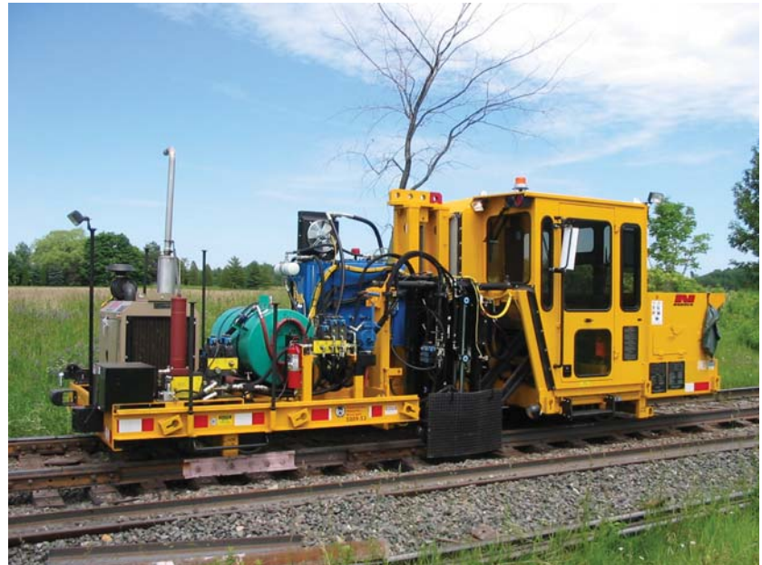
CX Hammer - Post Rebuild
