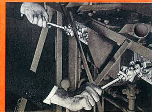
With one lever up, the other down, one ram moves upward and the other ram downward.
