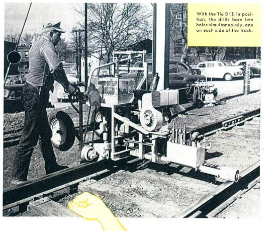
hoses which are long enough to reach spikes at either rail. The power plant is mounted on a frame equipped with a rubber tired wheel like a wheelbarrow for off-track movement. It has two ball bearing, double flanged rollers and outrigger for movement on the track. The power plant is a piston type hydraulic pump of the type used successfully for many years in the Nordberg Power Jack and Cribex. It is driven by a gasoline engine.
