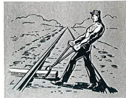
INSERTING TIES
