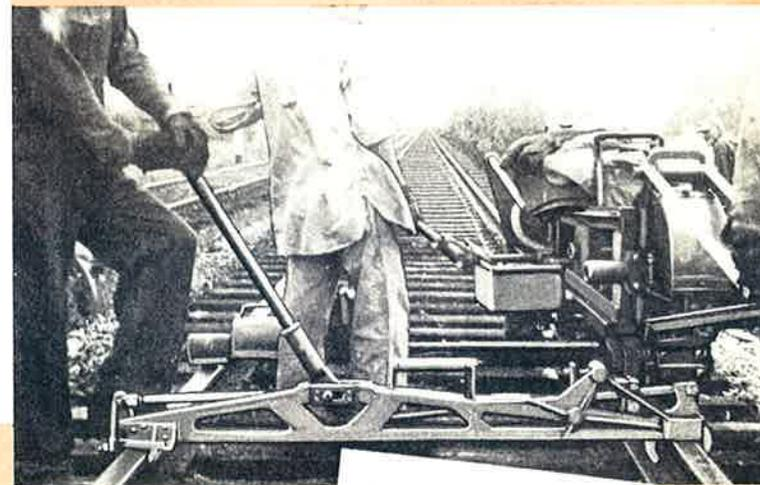
*Trakgager* holds rail in gage while gage spikes are driven with *Nordberg Spike Hammer*.
