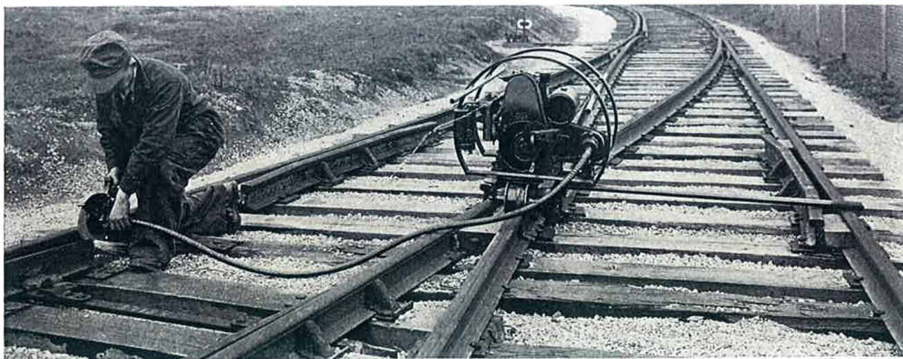
Grinding switch points and frogs is one of the uses to which the Cross Grinder can be put.
