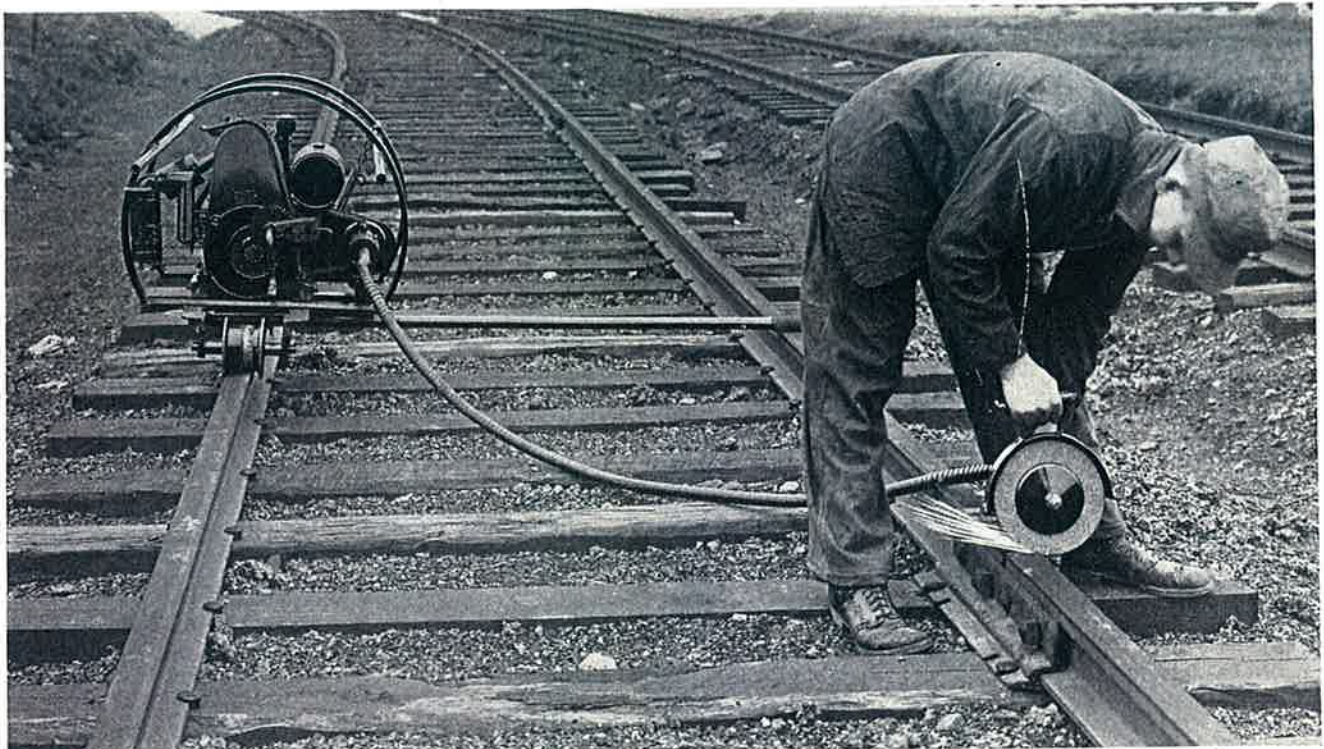
As the operator moves from joint to joint, the Grinder is rolled along on one rail. The 9 foot flexible shaft easily reaches either rail.
