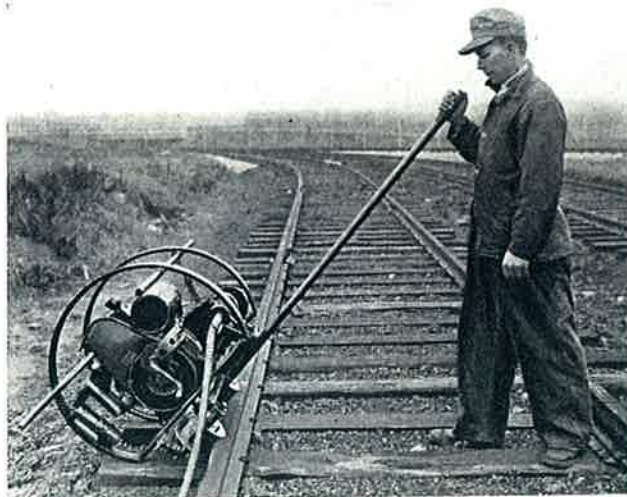
Should it be necessary to remove the Cross Grinder quickly in case of an approaching train, it is only necessary for the operator to raise the supporting bar and roll the machine off the track.
