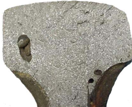
Thermite weld with slag entrapment
