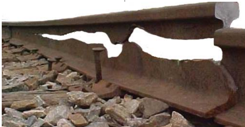
Web failure resulting from high residual stress.
