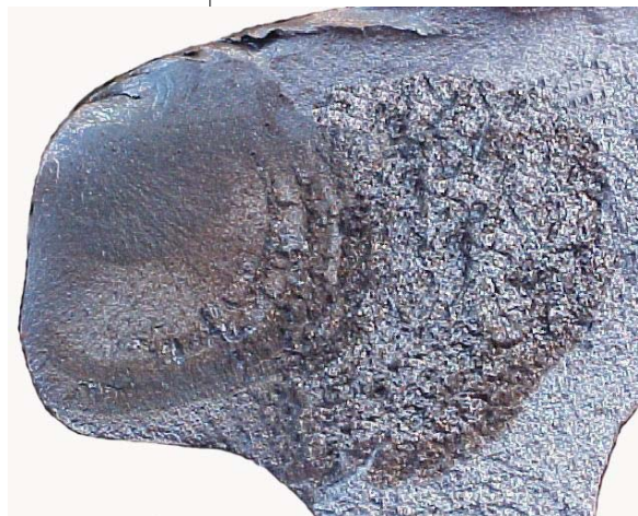
Detail Fracture from a Head Check
