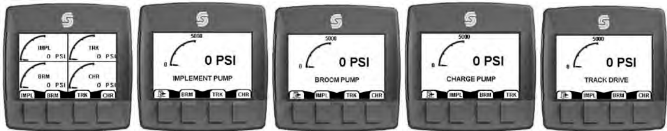
FIGURE 11. OPERATOR STATION CONTROLS PRESSURE SYSTEM DISPLAY GAUGE
